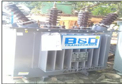
Gambar 2.1 Transformator distribusi 3 fasa
